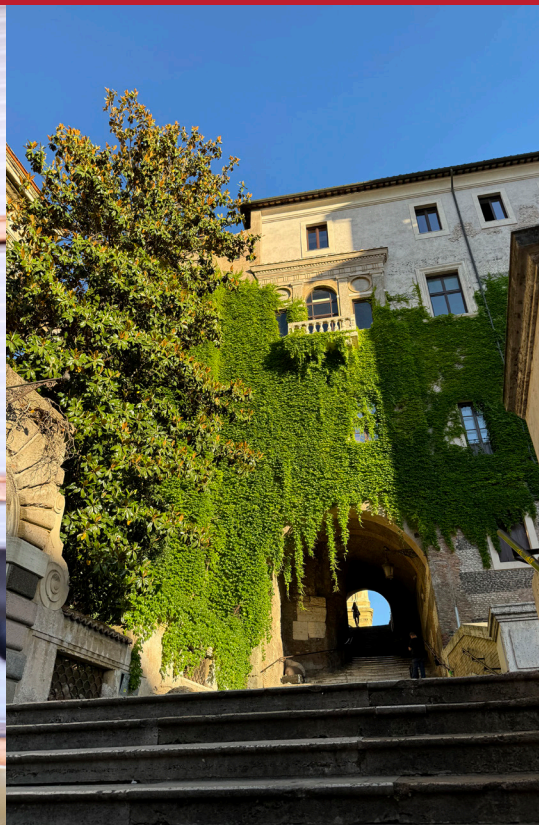
PLANT OVERGROWTH ON STEEP ROMAN STEPS
